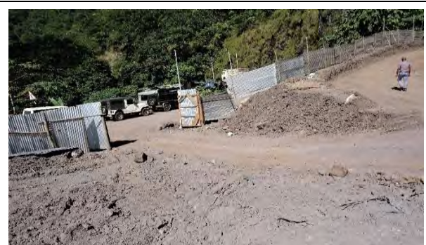
Dumping of topsoil along the roadside without providing any gullies/drainage channels at Mawlong area under DFO(T), Shillong
