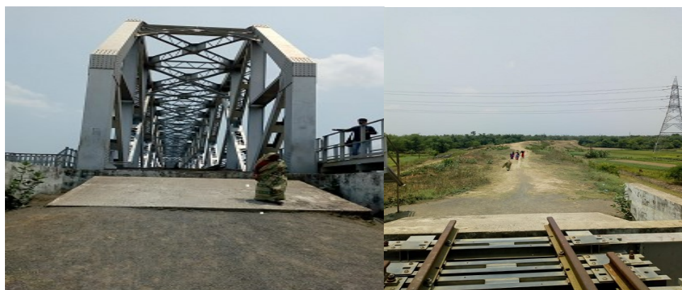
End of Railway Bridge over river Bhagirathi (Azimganj side)
