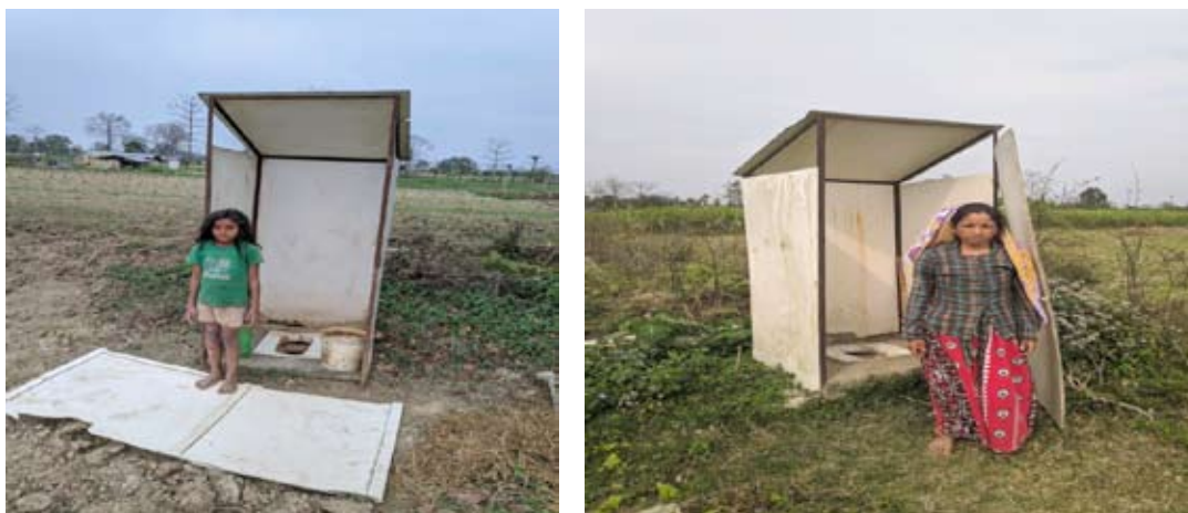
Dilapidated condition of the pre-fabricated toilets
