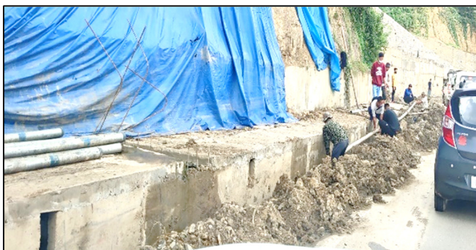
Digging of pits for laying of pipelines instead of using the duct.
