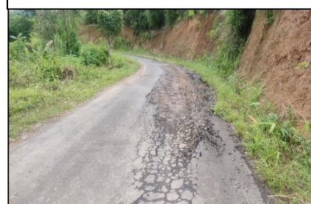
Photograph showing multiples potholes on the stretch of completed 9.5 Km
