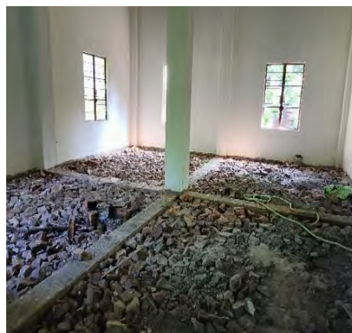
Incomplete New FPU
