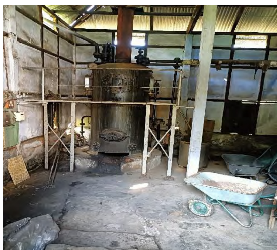
Condition of existing FPU
