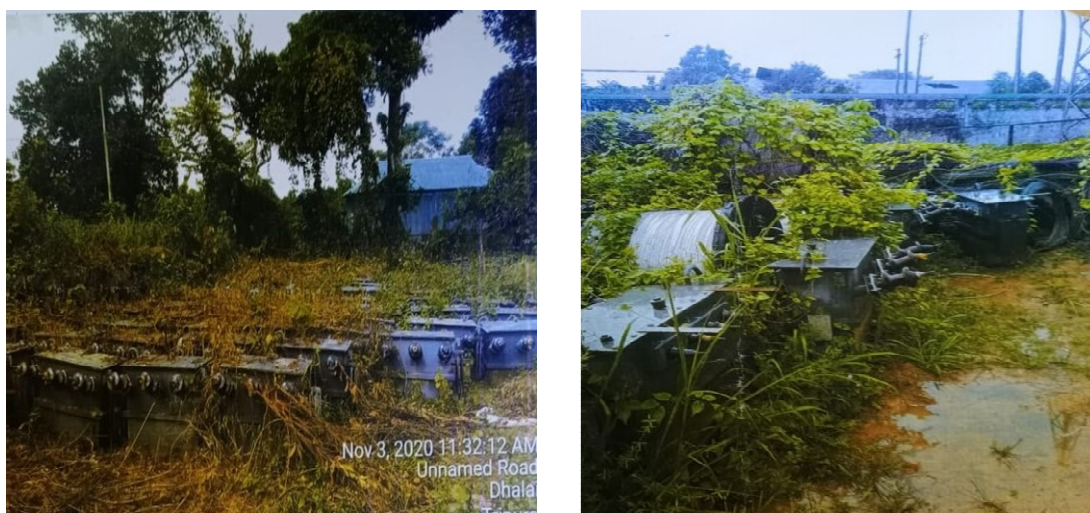
Transformers lying at open space, muddy surface, covered with bushes at Ambassa Store yard in Dhalai District
