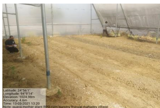
Tubular polyhouse lying idle (Ukhrul district)
