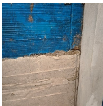
Cracks on ceiling of ground floor
