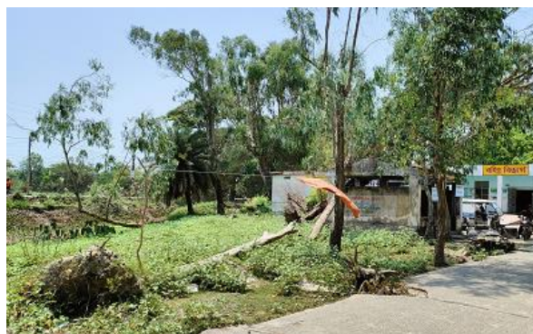
Picture 5.6: No boundary wall of Sandalerbill RH, Bashirhat (April 2022)
