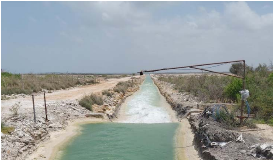
Figure 4.1: Treated wastewater being discharged through open channel at marine outfall point in Gulf of Kachchh at Mithapur
