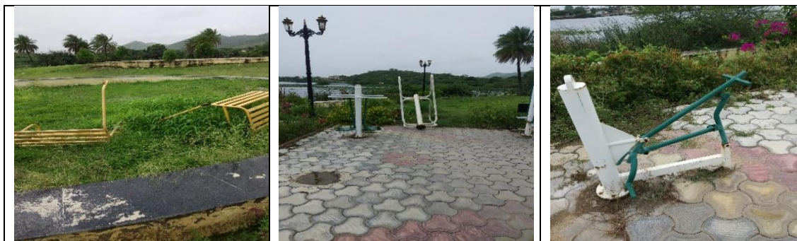
Images showing poor maintenance of installed equipment in garden (04.08.2021)
