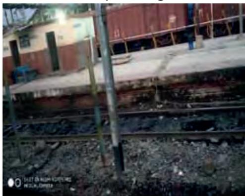
**Figure 4.3: Waste/water of public toilet damaging the track on Platform No. 04/05 at Gaya (ECR)**
