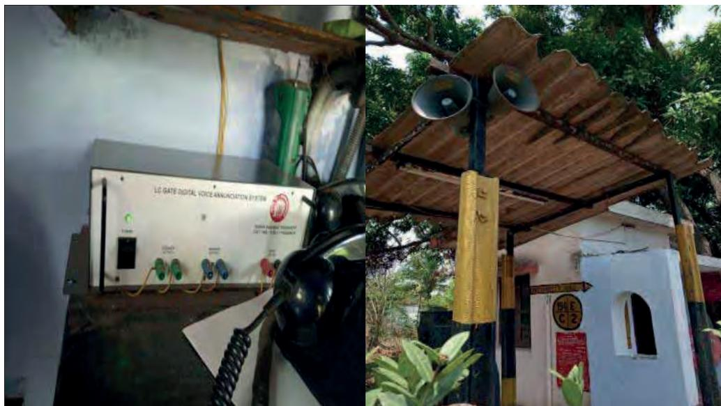
Figure 2.23: SR: Honey Bee Sound Device equipment installed at LC No. 154 (A line) between Walayar and Kanjikkode
