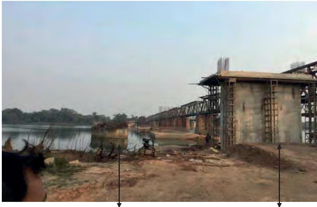
*Figure 3.10: Abandoned bridge constructed with Well foundation*
