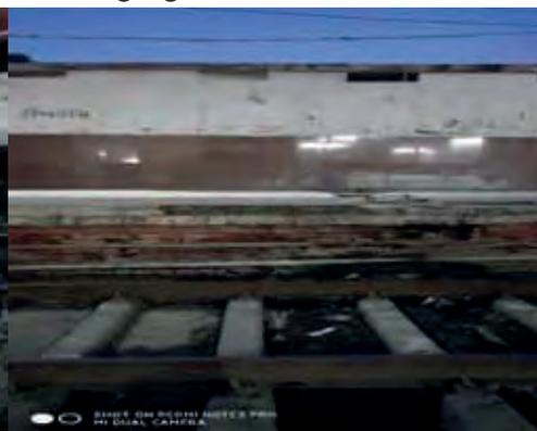
**Figure 4.4: Waste/water of public toilet damaging the track on Platform No. 02/03 at Gaya (ECR)**
