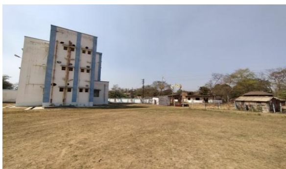
Pic 2.5.1: No boundary wall in Girls' Hostel (GH) of Khasjantal NIGS, Paschim Medinipur
