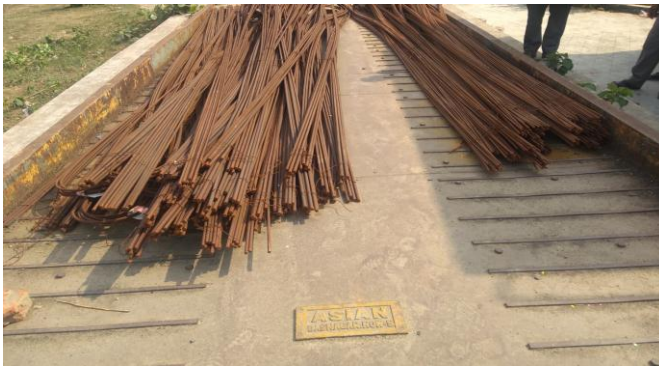
Pic 2.3.5: Construction materials being stacked on the unused Weigh Bridge platform at Tehatta KB Nadia
