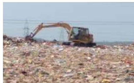
Photograph 9: Chain mounted dozer inside Bhuasuni dumping yard, BMC since June 2020
