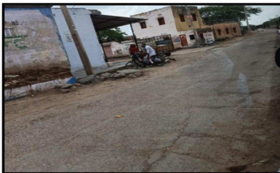
Image 4: Unconstructed stretches of the road
