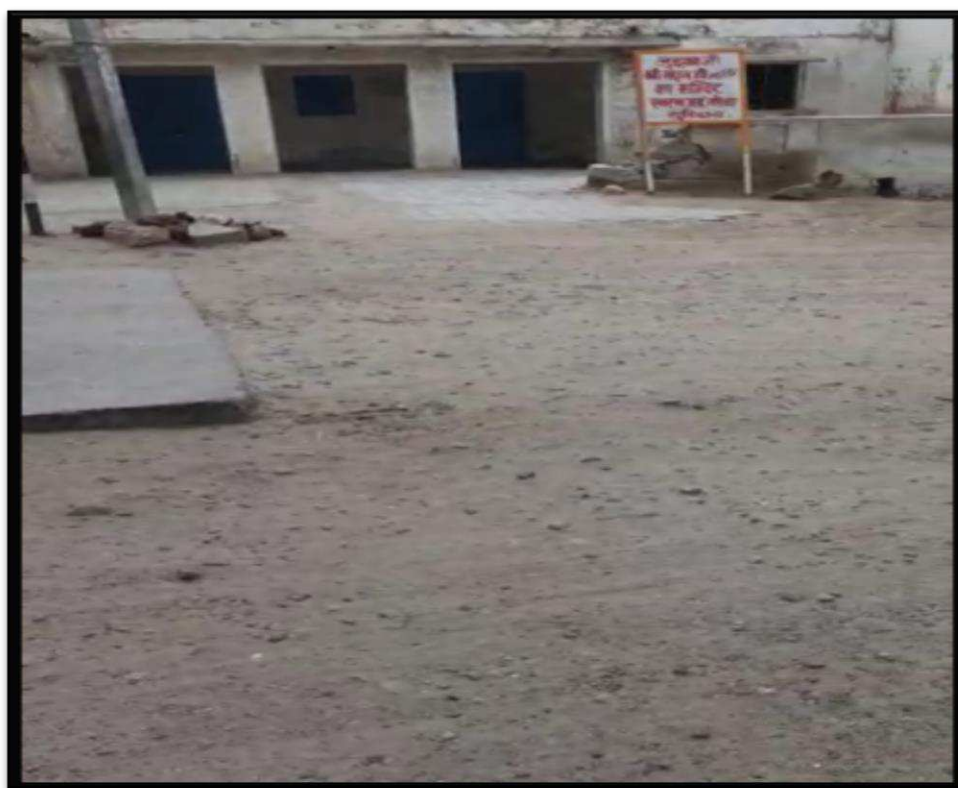
Image 3: Unconstructed stretches of the road
