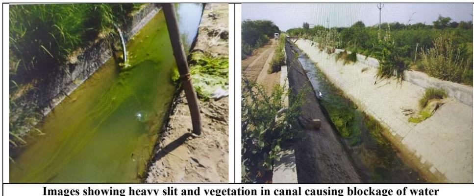
State Government stated (March 2021) that the work of removal of silt, etc. is carried out by WUAs from time to time, particularly before start of Rabi season. Reply is not tenable as heavy silt deposition, vegetation and algae were found during joint physical inspection.
