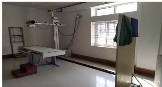
X-Ray room had a glass window which was adjacent to the parking area (February 2020)
