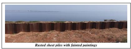
job worker for painting 32,694.19 sqm as of June 2021. In the JPI, conducted on 18 August 2021, Audit observed that exposed part of the sheet piles spreading over 2.76 kilometers were rusted and only light traces of paint were found with only two months of the work reported to have been executed. Further, the piling work had not yet been completed despite stipulated completion date of February 2021. However, the full amount of ₹58.20 lakh had been paid to the job workers.
