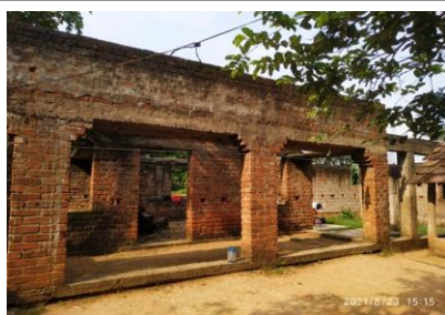
Incomplete Kitchen-cum- dining room at CCI, Mangalpur
