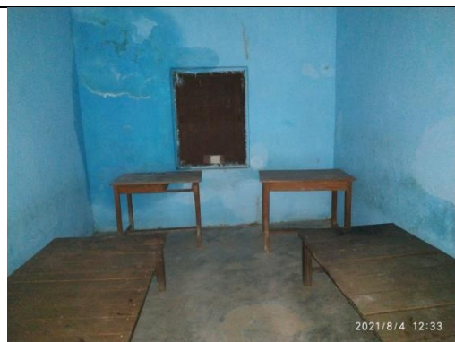
WWH at Olatpur: Two bedded room. Sidewall is soaking and needed renovation
