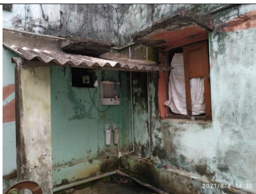
Water purifier fitted in the courtyard. The window of the kitchen is broken and required immediate repairs
