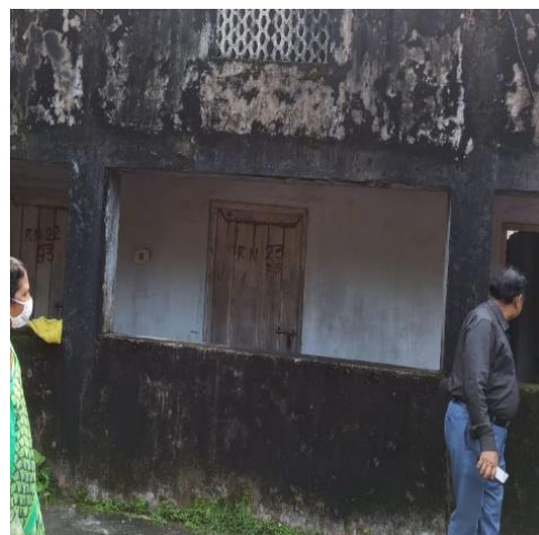
Outer condition of the first floor
