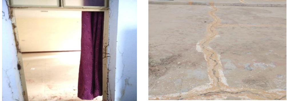
Termite hit door in Museum building
