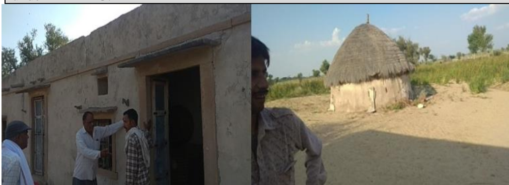
Pucca house of the beneficiary with more than three rooms.
