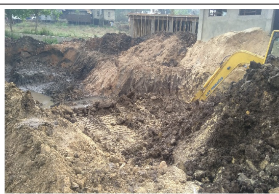
Slow progress of construction of the Farmers' Market at Mawryngkneng, East Khasi Hills.
