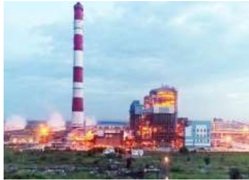
Singareni Thermal Power Plant
