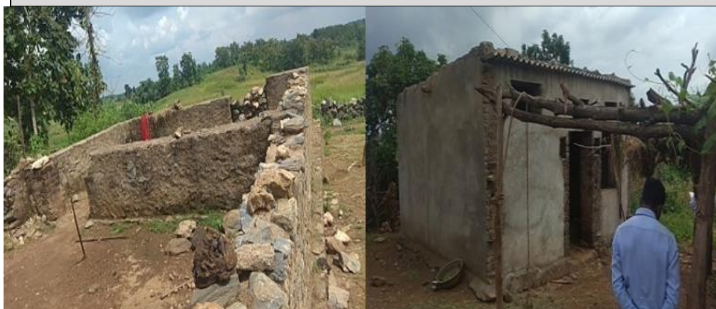
Date of Physical verification: 26 September 2019
