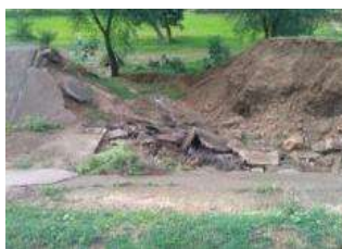
Breach in embankment near Phukujodi village
