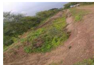
Sliding & silting of lining near Phukujodi village
