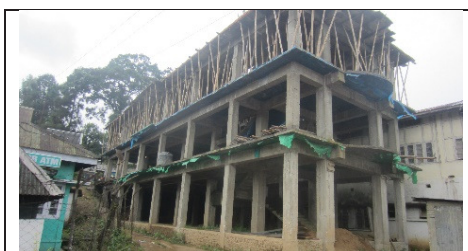
Photograph showing stage of completion of Court complex at Tuensang
