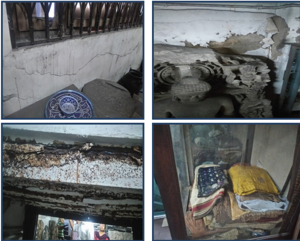
Reserve store – Roof with rust and termite, Artefacts on ground, Fabric bundled and stacked
