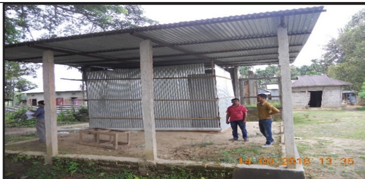
Photograph 5.2.1: Construction of Community hall at Dasami Ghat under 28- Teliamura AC
