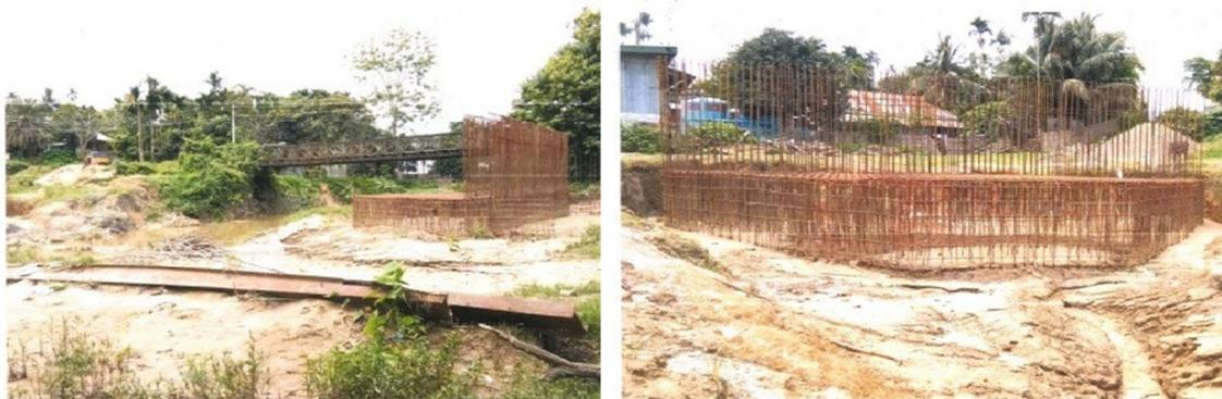
**Photographs 4.4.7 & 4.4.8 taken on 30-07-2018: Construction of RCC bridge over Gandacherra on the road from Gandacherra to Raishyabari at Ch. 1.00 km**
