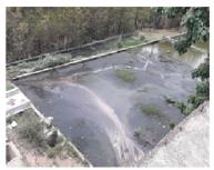
Uncovered sludge drying beds inundated/ overflowing with water at STP, Shamti, Solan (05 June 2018)
