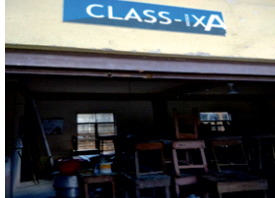
Class Room constructed at Government KVM High School being used as store room
