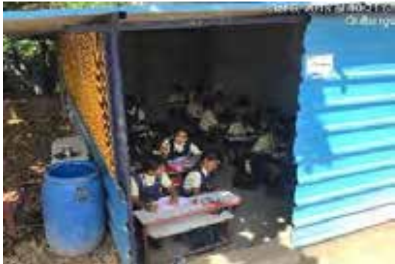
Sri Sai Central High School, Kalaburagi functioning in a structure made of asbestos sheet
