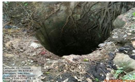
Pic. 14: Para No. 7.1.1: Improper closure of Dalmiya UG pit at ECL closed prior to nationalisation
