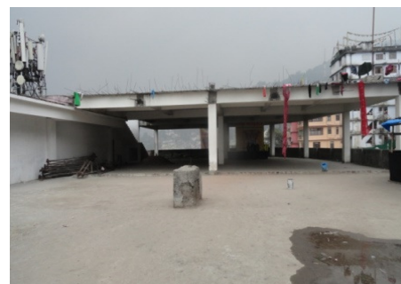
Idle and incomplete structure for Call Centre
