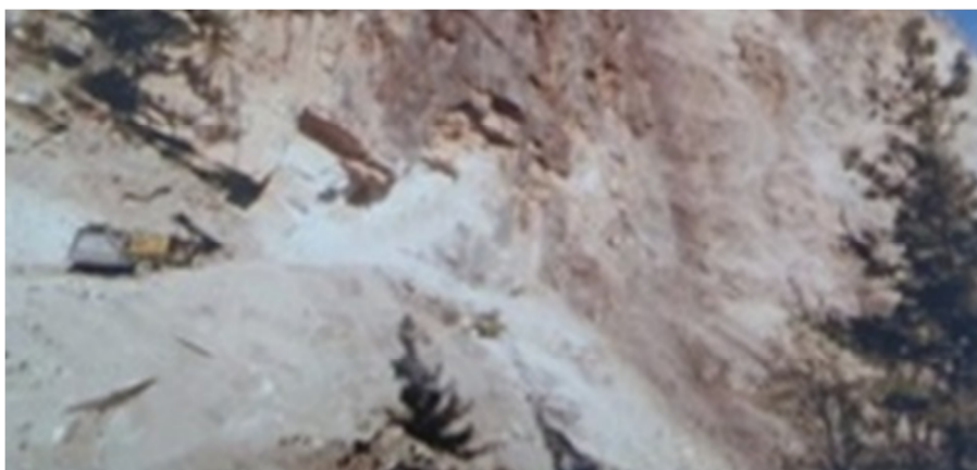
Dhandol to Kashapat road stretch from 11.300 kms to 11.375 kms
