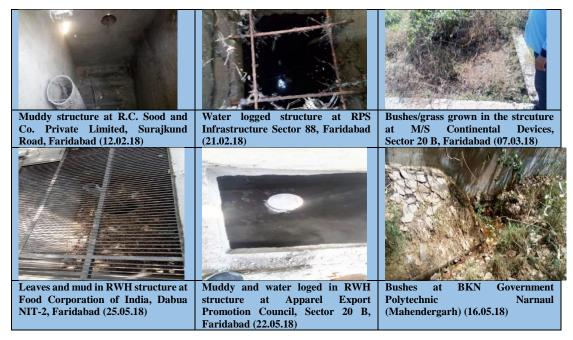
As is evident from above photographs, the structures were muddy/water logged and filled with garbage, plastic bottles, grass/bushes, etc. which hampers the seepage of rain water through RWHs for augmentation of ground water level in the area.
