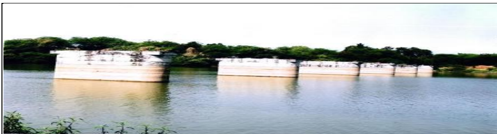
Source:- Photo of the incomplete high level bridge taken in February 2018
