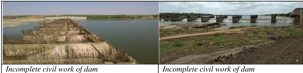
Incomplete civil work of dam
