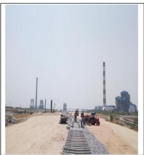
Picture No. 2.1.2:Track laying in RSMY works
