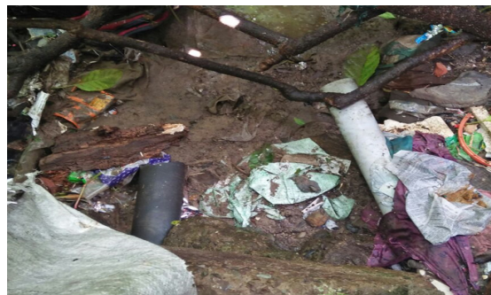
Sewage pipes being discharged into the open by households in Dharamsala (24 May 2018)
