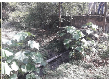
Leakage from Dholra Septic Tank, Bilaspur flowing into Govind Sagar (26.04.2018)
