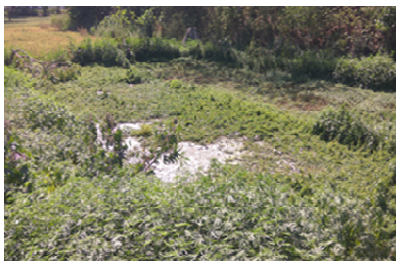
Overflowing septic tank at Una (Zone-C) (29.03.2018)
