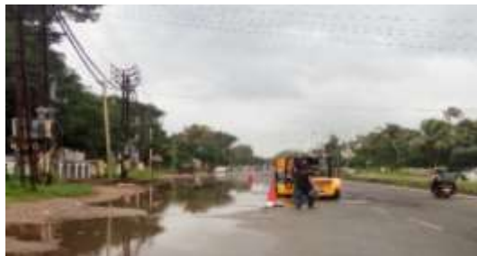
Picture 8: Lack of drainage caused water logging and potholes, reducing the width of carriageway in NH 66 (photo taken on 14/08/2018)
