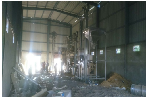
Photograph 2.2.1: Cleaning and Grading unit – Machinery under installation in Sedam, Kalaburagi District.
