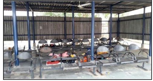
Figure 9: Broken chairs at waiting hall in SKK ISBT
