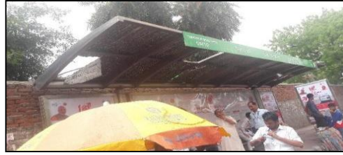
Figure 15: BQS with broken roof
