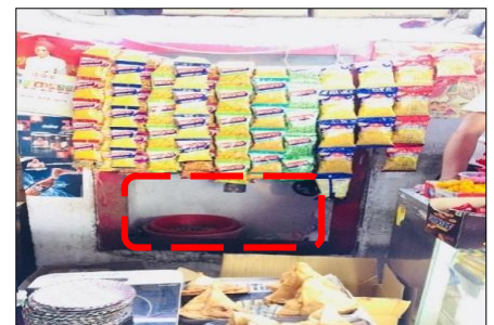
Figure 5: Fire Hydrants blocked by Kiosks
