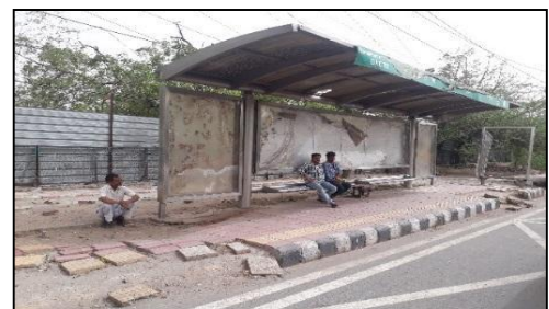
Figure 14: Poorly maintained BQSS with broken flooring
