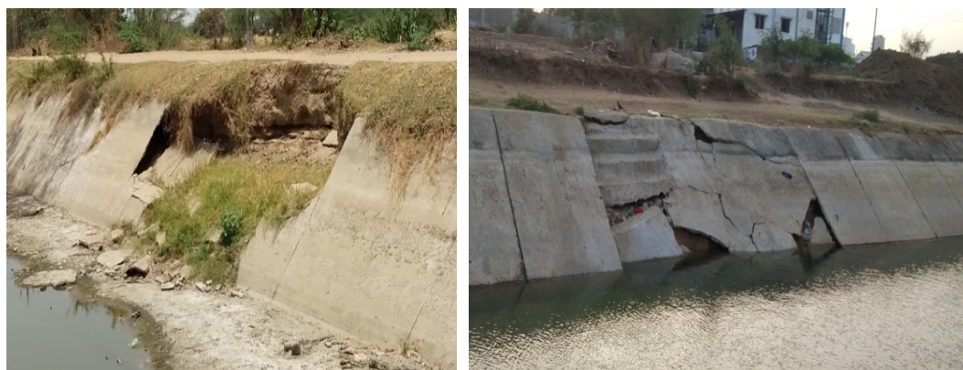
Damaged lining of Moti Fatewadi Canal at ch 10,670 m, Ahmedabad (2 June 2018) Damaged lining at ch 45,370 m of URBCI, Ankleshwar (15 May 2018)
