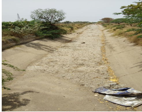
Siltation in extended canal of MFC at ch 10,670 m, Ahmedabad (2 June 2018)
