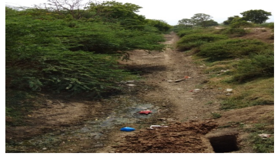
Vegetation in NFC at ch 100-500 m of Fatewadi Canal System, Ahmedabad (2 June 2018)
