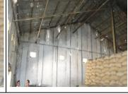
Photograph 1.2.2 and 1.2.3: Rain water accumulating inside the godown at Kichha (Udham Singh Nagar) because of damaged roof
