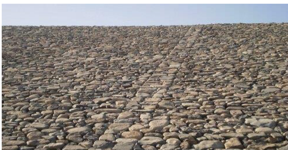
Figure 3.6 : Image of Loose Boulder Pitching
