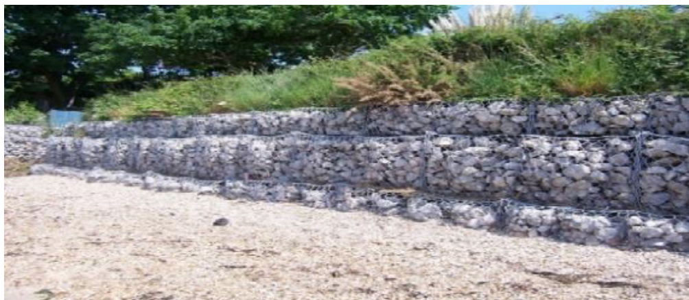
Figure 3.5 : Image of Boulder Pitching in sausage crate
