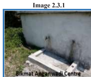
Empty Water Tank
