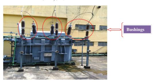
The Y phase bushing of GT of Unit II burst on 18 June 2015 leading to immediate shut down of the unit. A used reconditioned bushing that was installed on 28 July 2015, also burst after four hours of operation, along with the remaining two bushings (in phases R and B), leading to Unit II shutting down again.
