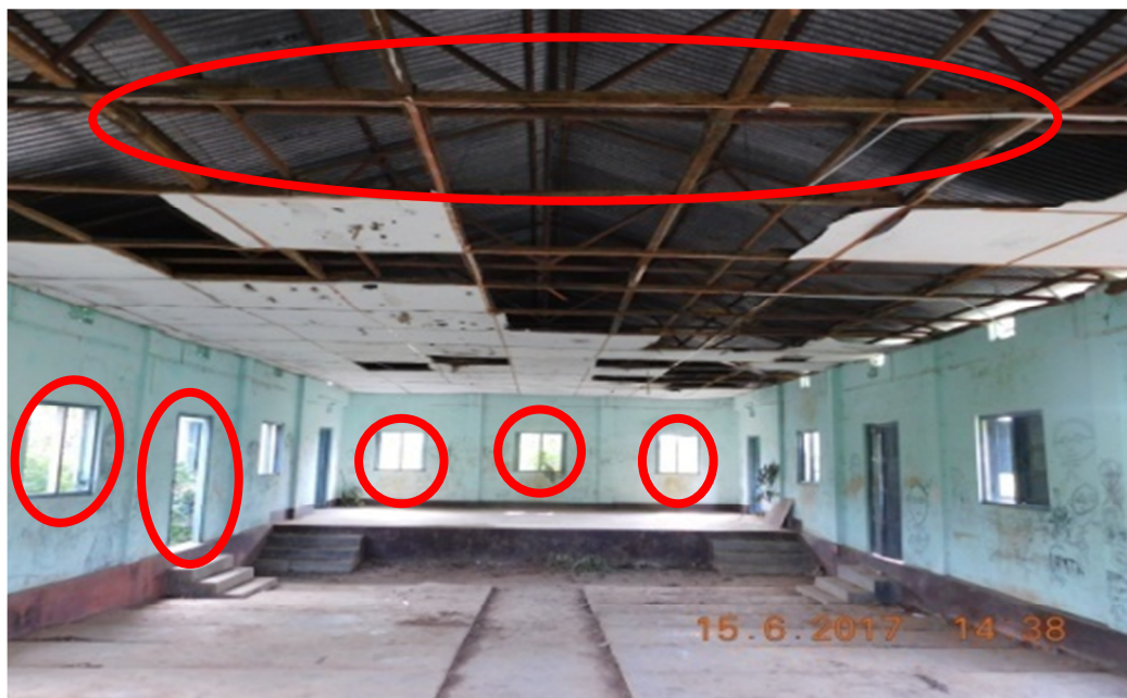
Photograph 4.3.11: Dilapidated condition of the community hall with broken doors, windows and ceiling
