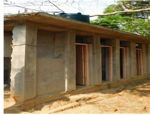
Photograph 4.3.4: Construction of toilet (three unit), bathroom (one unit) with Ordinary Hand Pump (OHP) at Daigyabari
