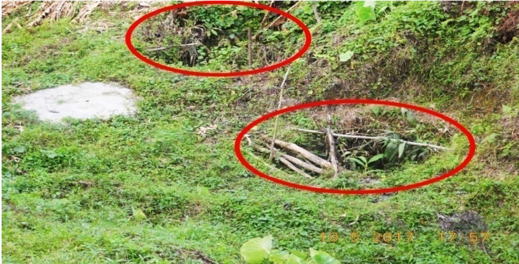
Photograph 4.3.1: Construction of ring well/deep tube well with motor pump (stand by pump) including laying of pipe water storage tanks and iron removal filtration plant at Border Out Post (BOP), Khasiabasti.
