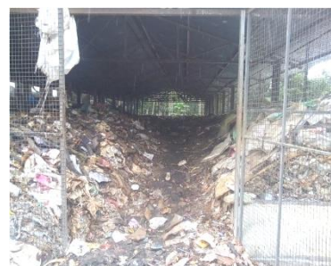
Exhibit No. 2: Waste remaining untreated in the treatment plant at Erumeli (04 August 2017)
