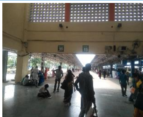
Fig.4.8 Two new platforms (No.15 and 16) at MASS
